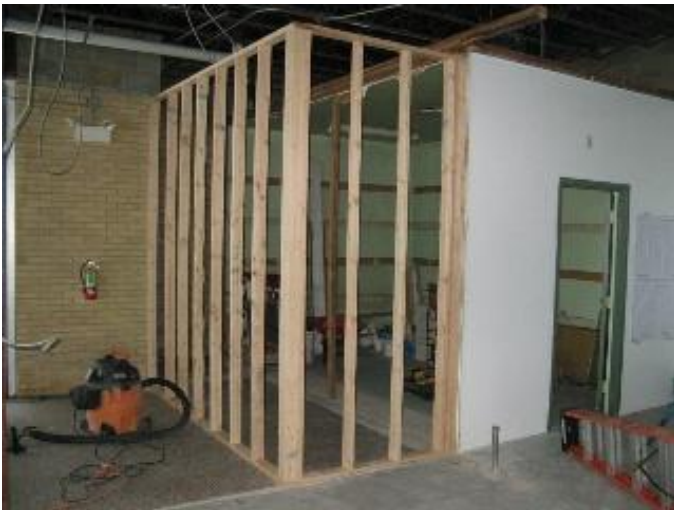
Framing begins on the new storage room. (Photo by Frank Warner)
