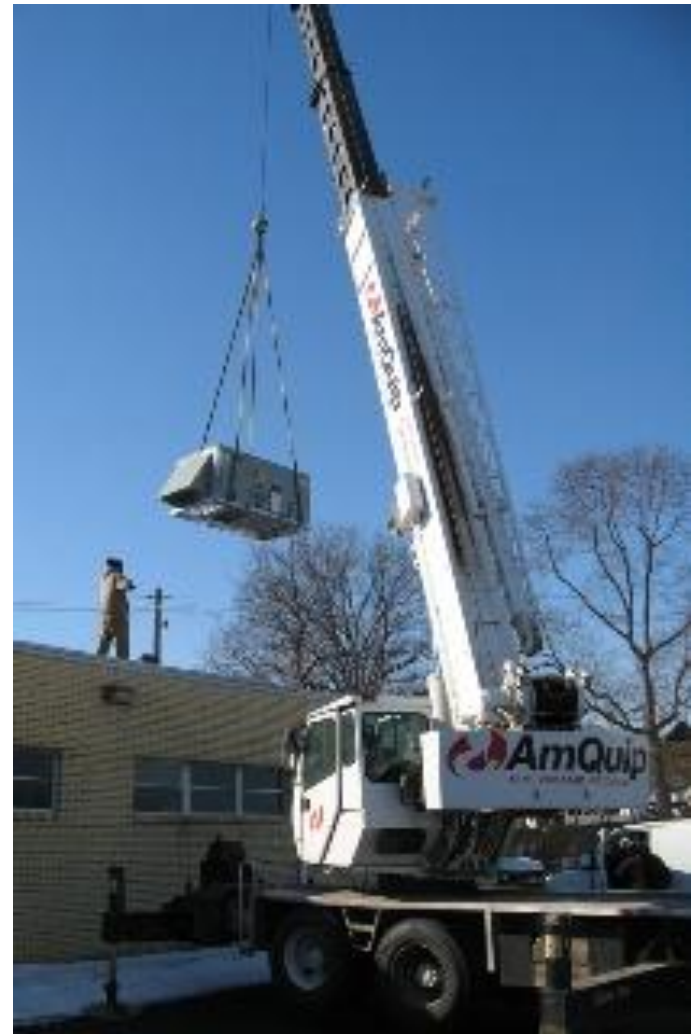
The new HVAC unit is placed. (Photo by Frank Warner)
