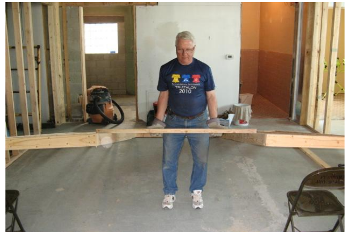
Bill Mattis lifts one on the partitions. (Photo by Frank Warner)
