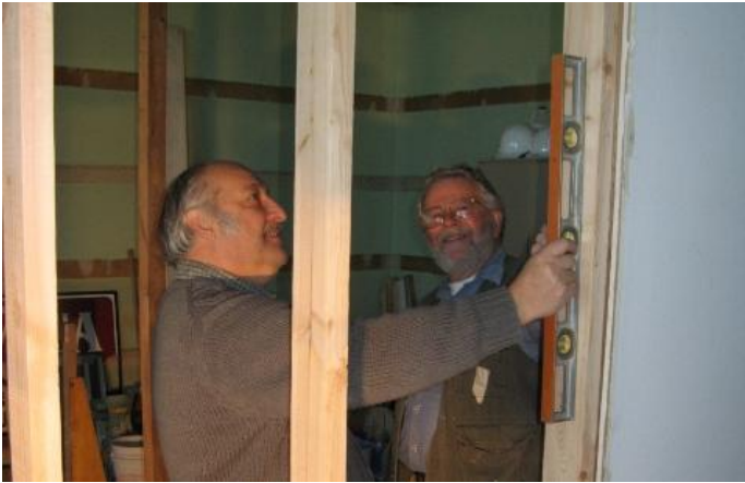
Pete Santucci and Doug Klieger ensure the studs are straight. (Photo by Frank Warner)
