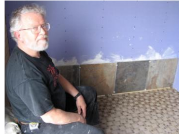
Doug Klieger sets the first tiles in the vestibule. (Photo by Frank Warner)
