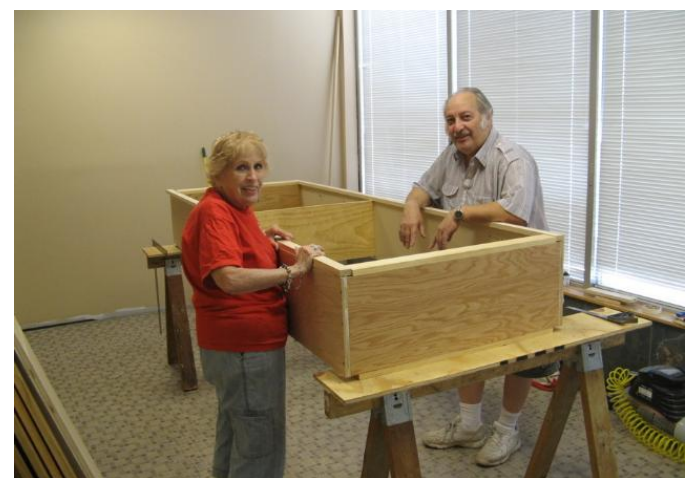
(Top left) Bill Mattis and our electrician, Jeff, place the final light fixture in the jewelry room. (Top right) Pam Wingrod and Lola Fields install ceiling tiles. (Bottom) Betty Margerum and Pete Santucci construct a book case for the library. (Photos by Frank Warner)
