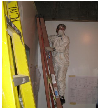
(Left) Lola Fields installs ceiling insulation. (Right) The inner vestibule door is installed. (Photos by Frank Warner)
