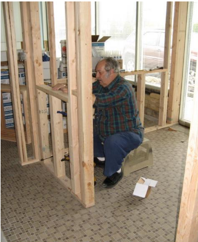
Pete Santucci works in the vestibule. (Photo by Frank Warner)
