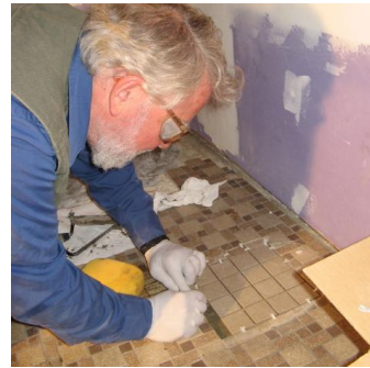
(Left) Doug Klieger patches the bathroom floor tile. (Right) Joe Pizzirusso primes the storage room walls. (Photos by Frank Warner)
