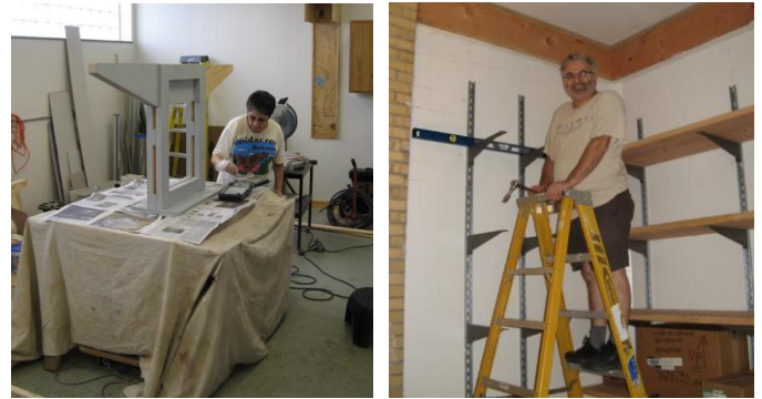
(Left) Pam Wingrod paints jewelry bench supports. (Right) John Chickadel installs shelving in the new storage shed. (Photos by Frank Warner)
